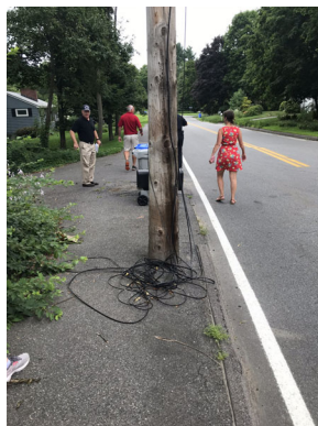
Exposed telephone wires along Woodland Street sidewalk
