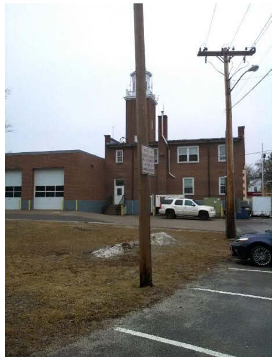
Future Home of Holliston's Electric Vehicle Fleet
