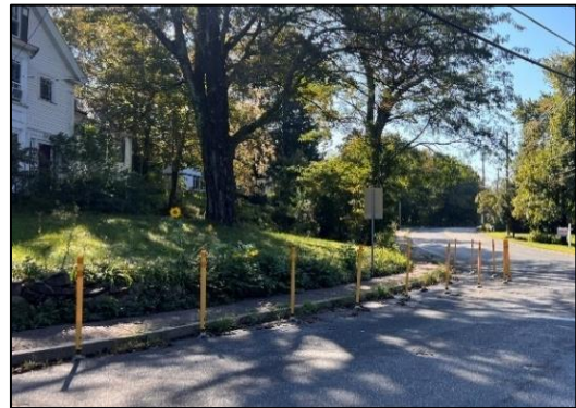
Photo 4. Tapered delineator along Franklin Street to slow vehicles down
