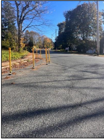
Photo 11. Sight distance looking left (south) from Franklin Street (southbound)
