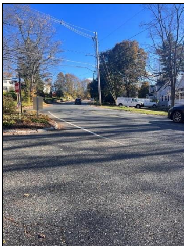
Photo 13. Sight distance looking left (south) from Franklin Street (westbound)
