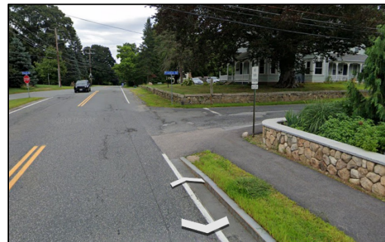
Photo 2. Intersection of Central Street at Franklin Street
