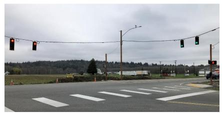
Photograph 11: Temporary Traffic Signals (Span Wire Mounted)
