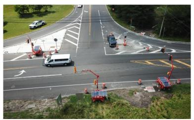
Photograph 10: Temporary Traffic Signals (Trailer Mounted)
