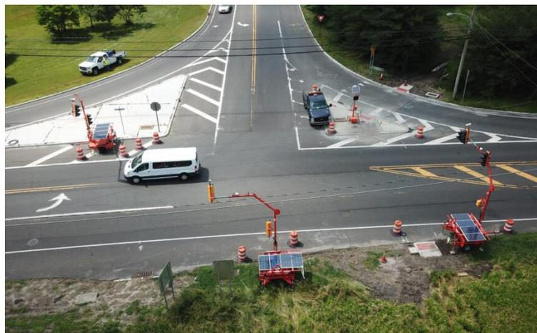
*Photograph 10: Temporary Traffic Signals (Trailer Mounted)*
