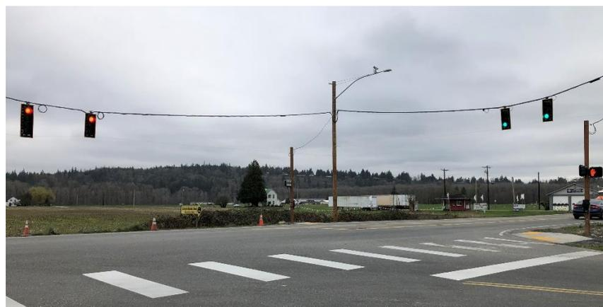
*Photograph 11: Temporary Traffic Signals (Span Wire Mounted)*
