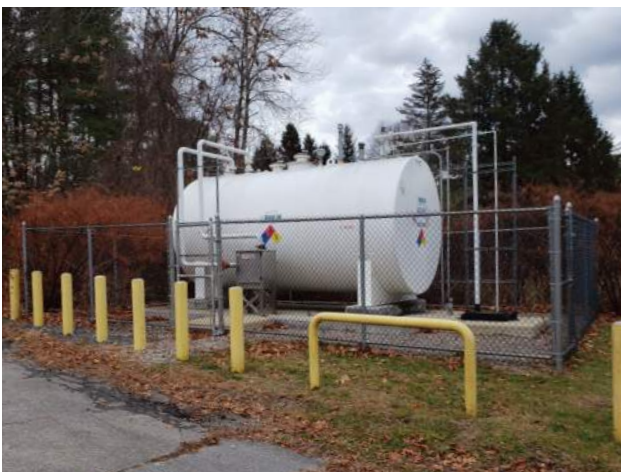
Above ground fuel storage tank
