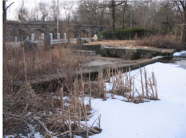
Image 2: Concrete walls at primary spillway approach
