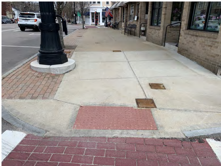
Ramp on Washington St with a landing slope over 3%
