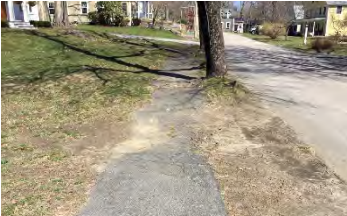
Example of tree root damage and a pinch point on Irving Place
