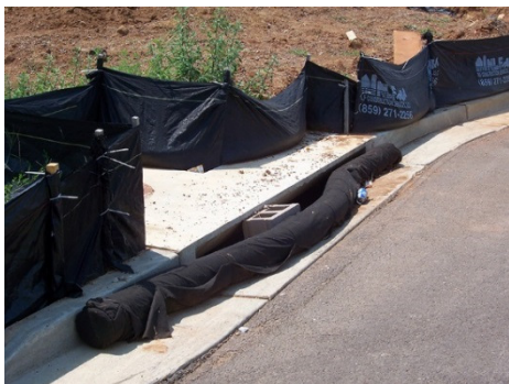
Typical filter bag inlet protection installation.
