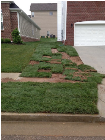
Sod installation failure. Sod needed staples. Photo credit:
