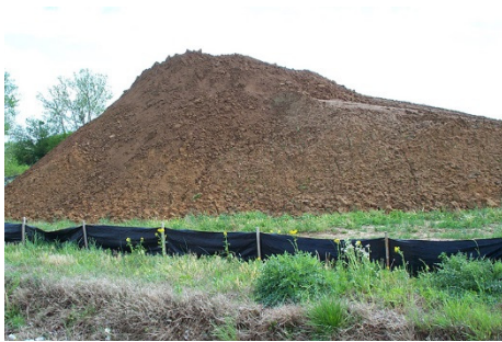
Silt fence around soil stockpile.
