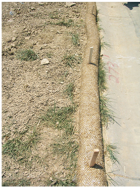
Drive stakes every 3-4 feet along the filter log.
