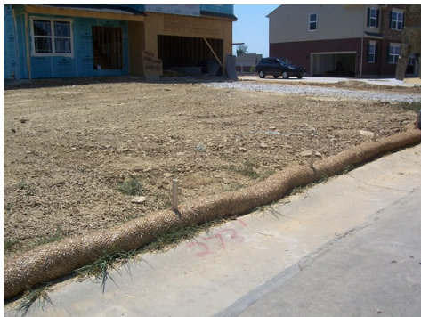
Make sure filter log stakes are spaced to prevent undercutting or bypasses. Leave stake tops extended along sections to prevent drive-overs.
