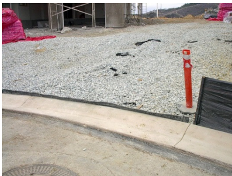
Good application of rock exit pad. Note short section of material against curb that is keeping rock from leaving site.
