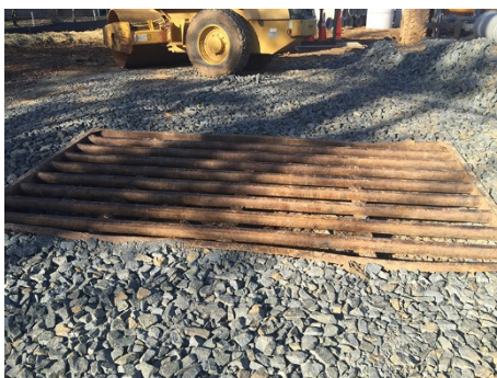
Rumble pad construction exit
