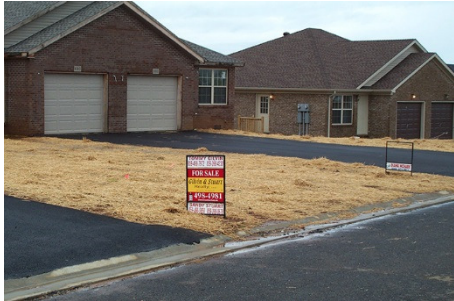
Straw mulch can be used to both prevent erosion and minimize dust from a site. Photo credit: Barry Tanning, Tetra Tech.
