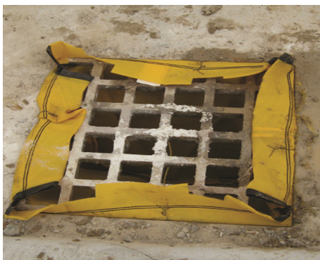
Typical filter bag inlet protection
