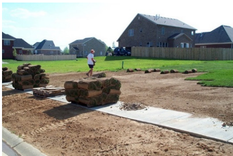
Photo of sod being installed at a residential site. Photo credit:
