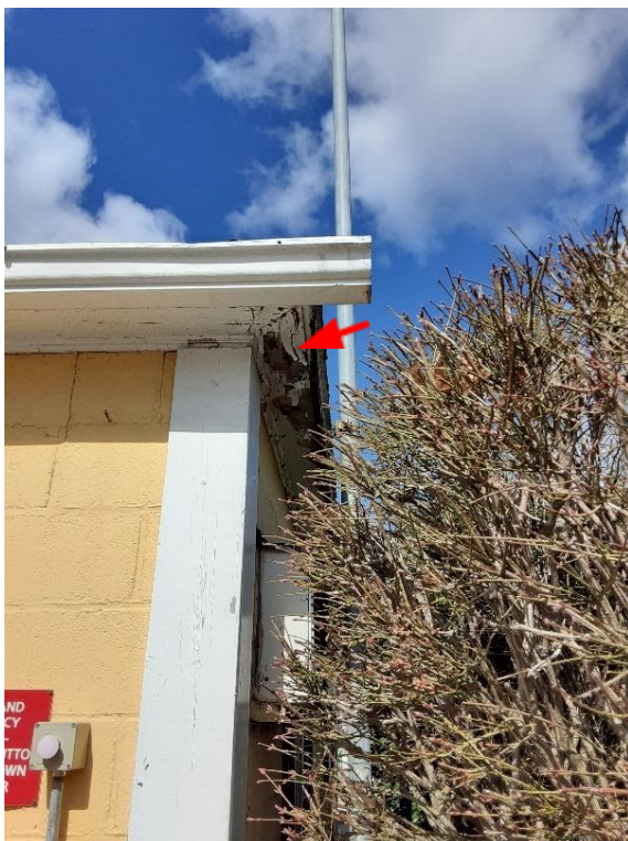
Damaged Soffit and block walls (Office/admin side)
