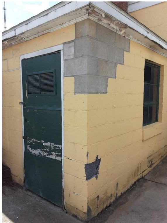
Damaged Soffit and block walls (Office/admin side)
