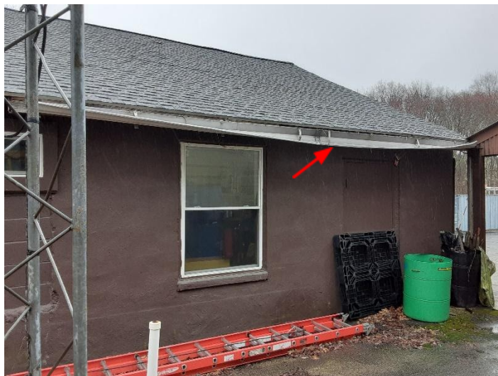
Southwest of Office/Admin building (damaged gutter)
