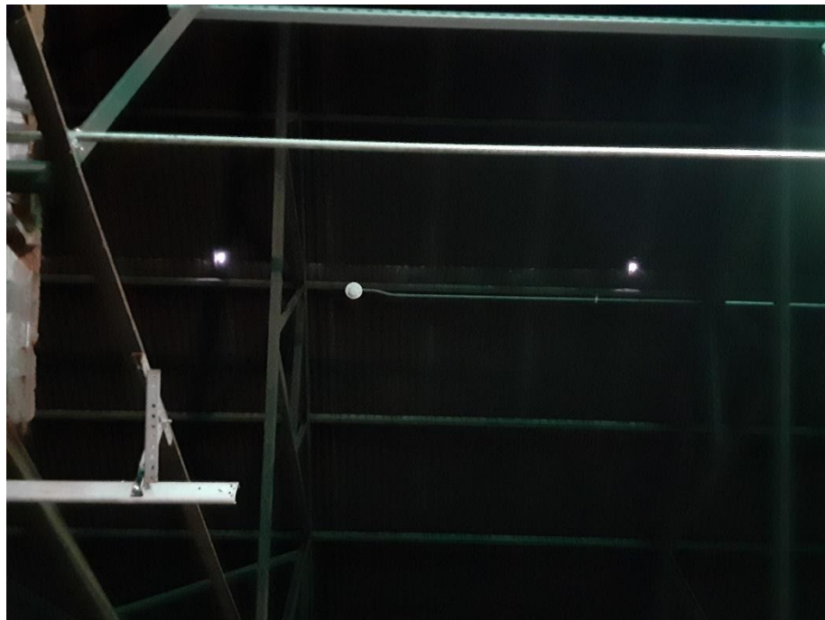
Additional holes in roof
