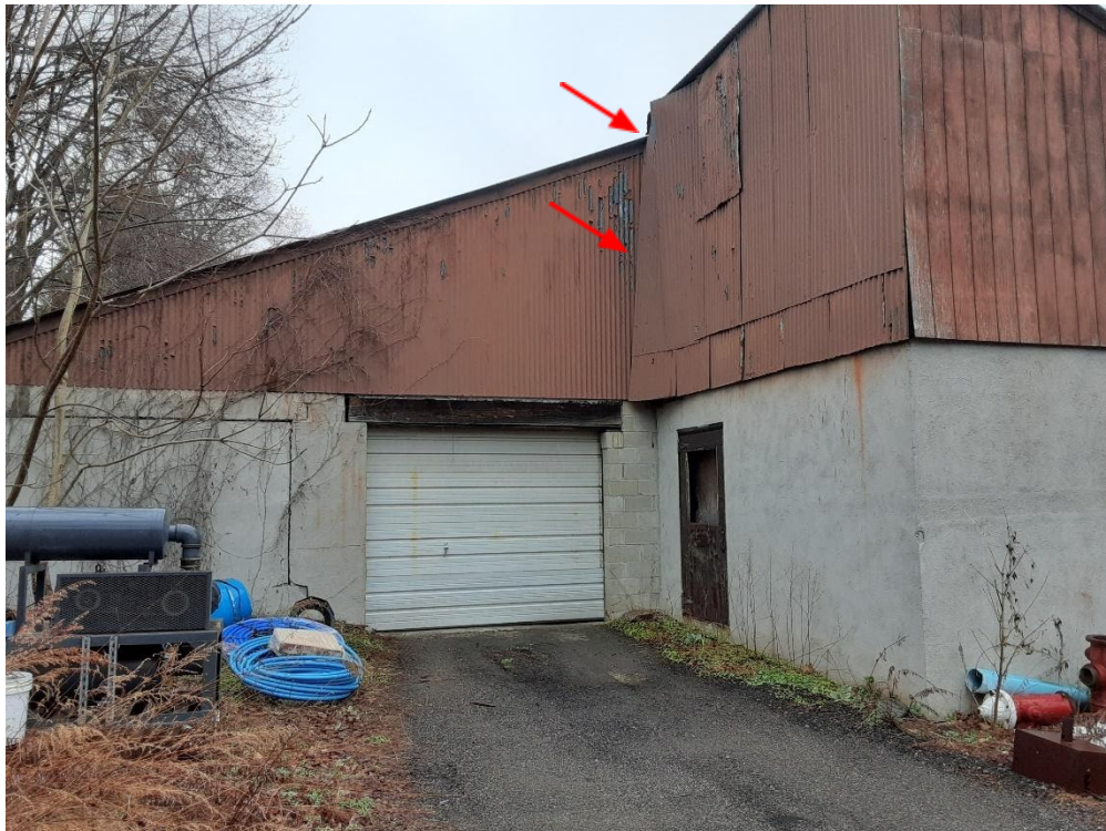
Rear of Vehicle Storage building (Arrow -siding pulling off)
