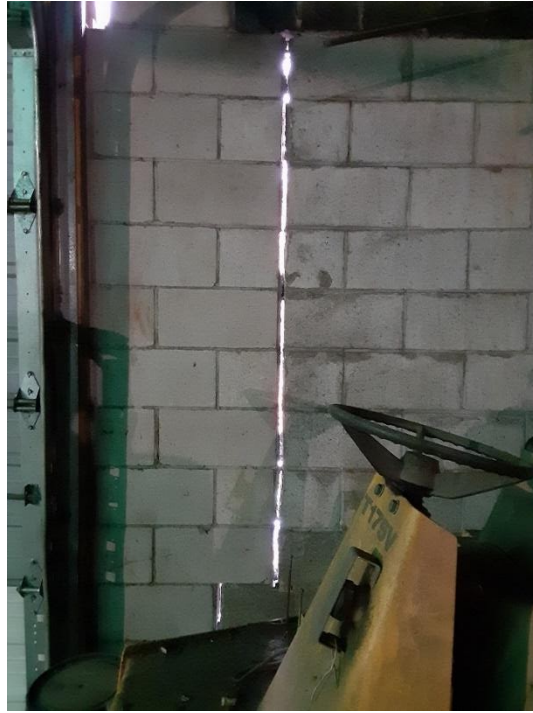
Large crack in wall
