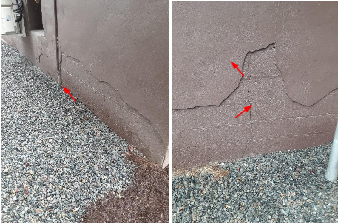
Damaged Stucco Office/Admin building
