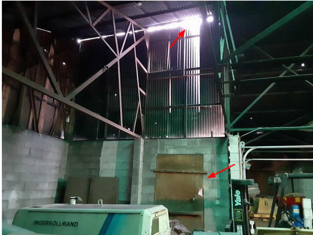
Inside view of failed siding and blocked door
